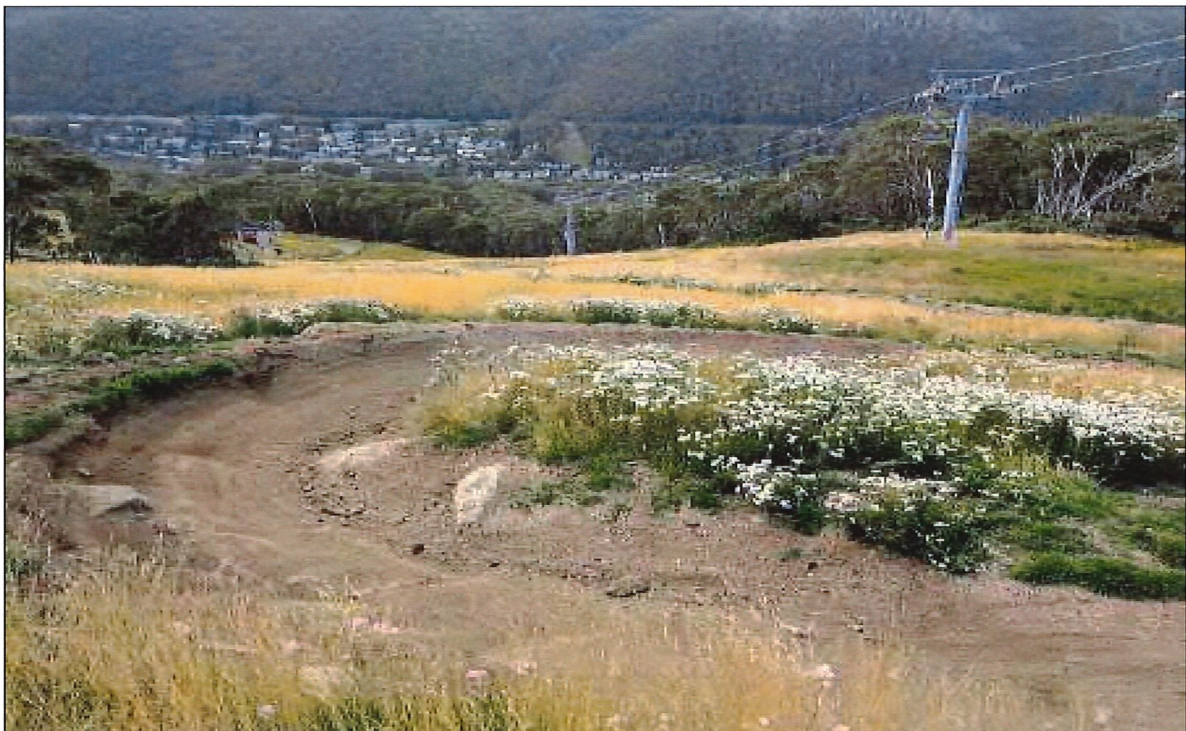
Figure 2: Example of an existing corner (berm) that is to be relocated off the ski run into existing tree islands or native vegetation (Source: Applicant's SEE)
